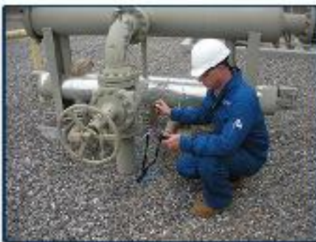
TP EUROPE Leak detection/repair
