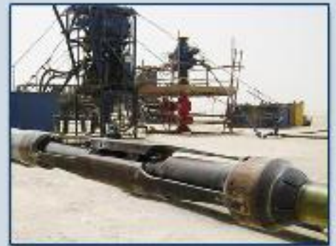
WWT - Drill pipe & casing
